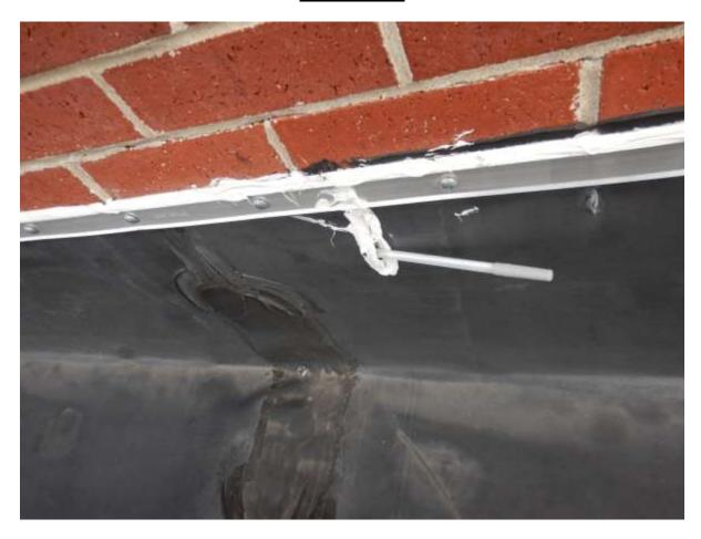
**CONDITION:** The base flashing is split at this location.
