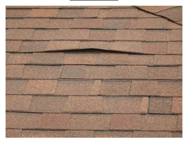
**CONDITION:** The shingle is raised from the protruding roofing nail.
