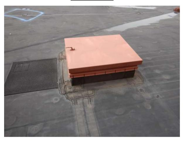
CONDITION: Use of the roof hatch presents a fall hazard. A safety rail system should be installed around this roof hatch.
