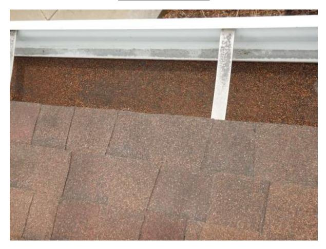
**CONDITION:** Granules are collecting in the gutter system.
