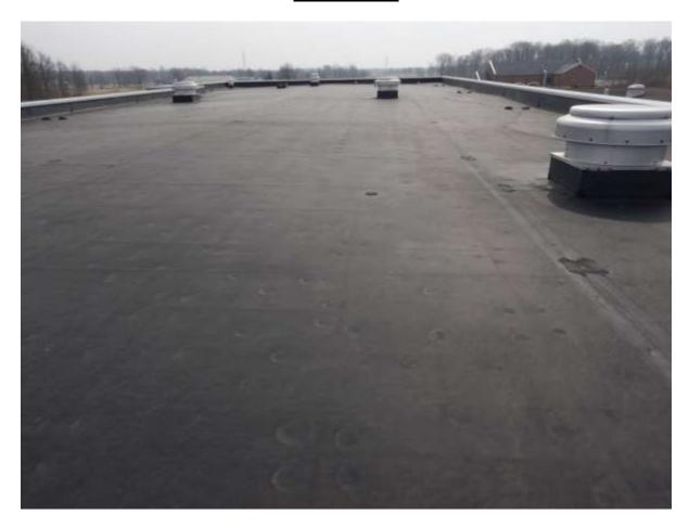
CONDITION: An overview of the Fully Adhered EPDM Roof System on Section A.
