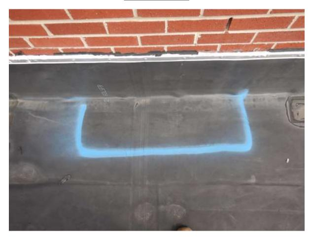
CONDITION: A view of wet substrate identified in the Infrared Moisture Roof Survey; no surface anomalies were identified in this area.
