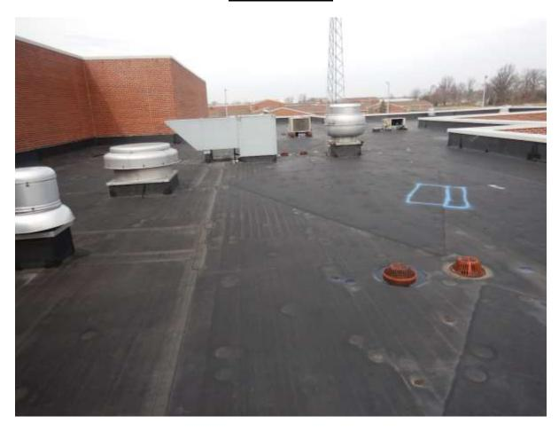
CONDITION: An overview of the Fully Adhered EPDM Roof System on Section B.
