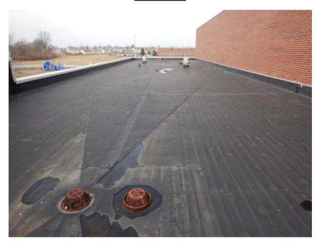
**CONDITION:** An overview of the Fully Adhered EPDM Roof System on Section C.
