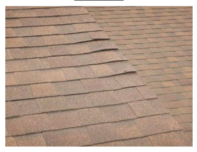
**CONDITION:** The shingles are raised at the perimeter edge.
