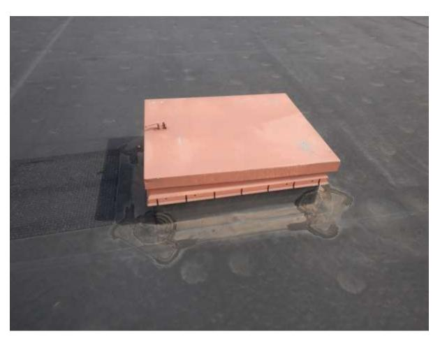
Use of the roof hatch presents a fall hazard. A safety rail system **CONDITION:**
