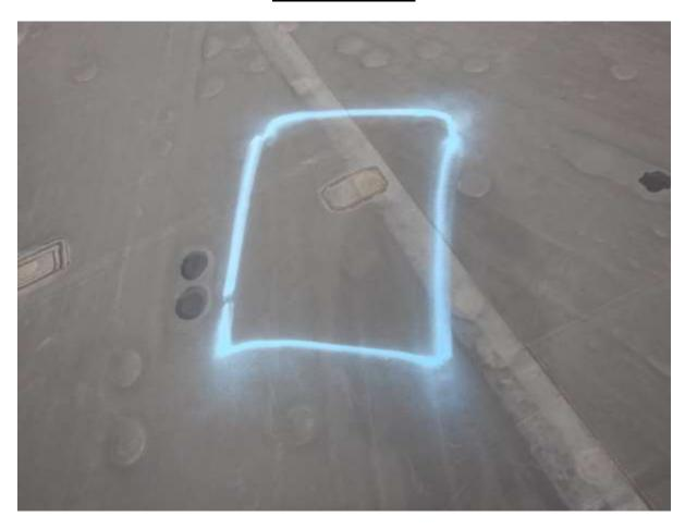
CONDITION: The field membrane is damaged within this area of wet substrate identified in the Infrared Roof Moisture Survey.
