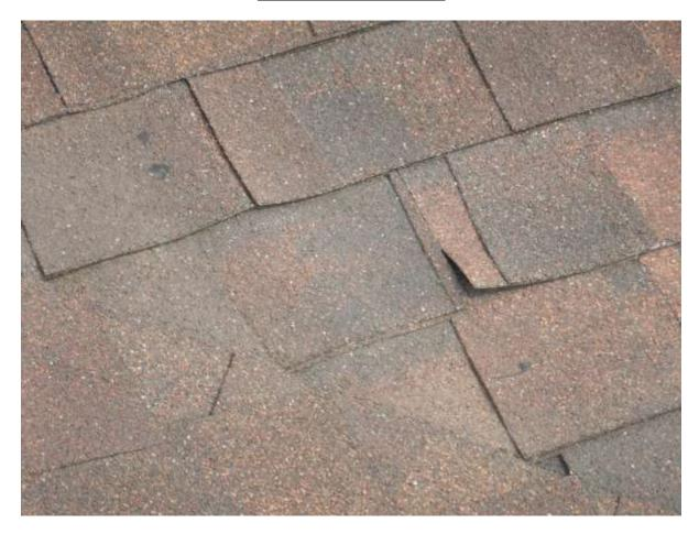
**CONDITION:** The shingles are buckled in this area.
