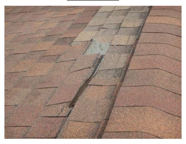
**CONDITION:** The Dimensional Shingles are damaged in this area.
