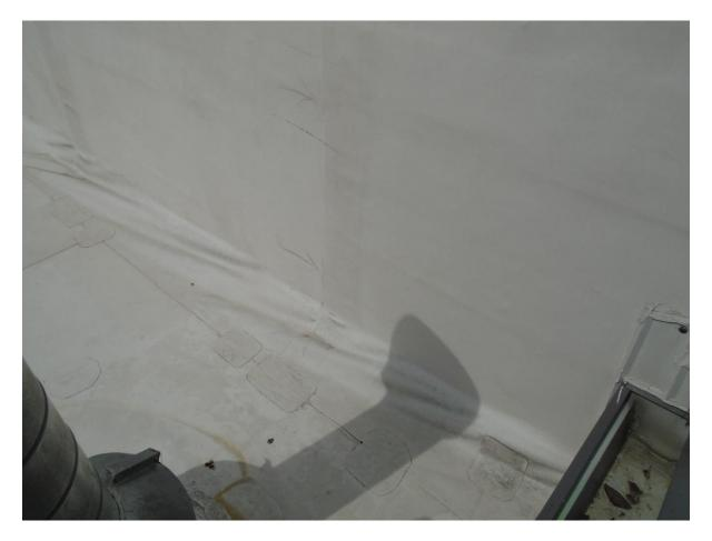
**CONDITION:** The membrane base flashing is racking in random locations.
