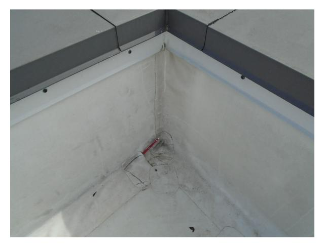
CONDITION: There is a void in the corner flashing at this location.
