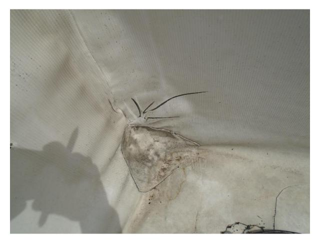
CONDITION: There is a void in the corner flashing at this location.
