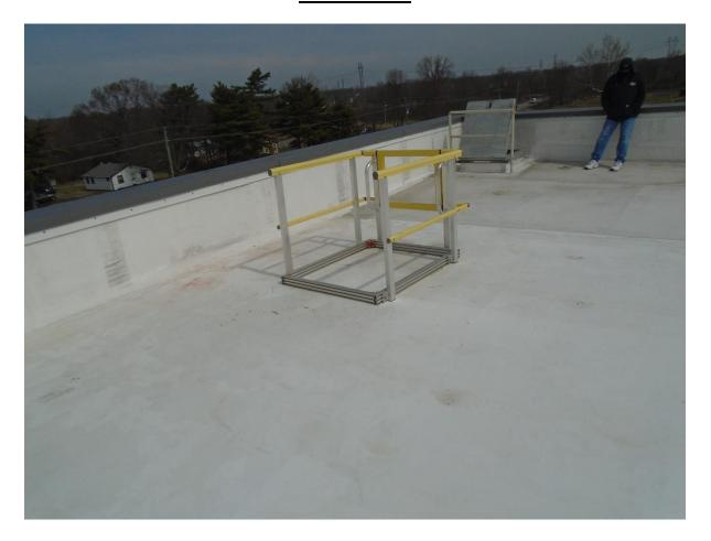
CONDITION: Another view of view of an uninstalled roof hatch safety surround. Nutec Roofing will be on site the week of April 12, 2021 to reinstall the gate as it was part of the roof repair scope of work they completed in 2020.
