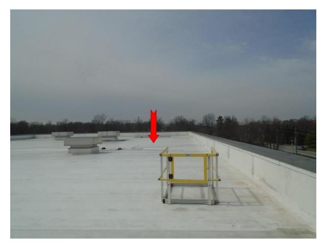
**CONDITION:** A view of wet substrate (*in the distance*) identified in the Infrared Roof Moisture Survey; one surface anomaly was identified in this area.
