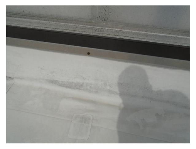
**CONDITION:** The membrane flashings are deteriorating at random locations.
