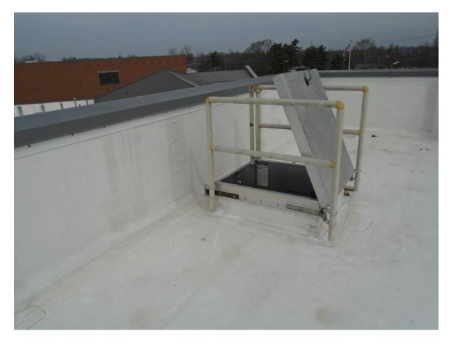
**CONDITION:** Use of the roof hatch presents a fall hazard. A safety operable rail system should be installed around this roof hatch.
