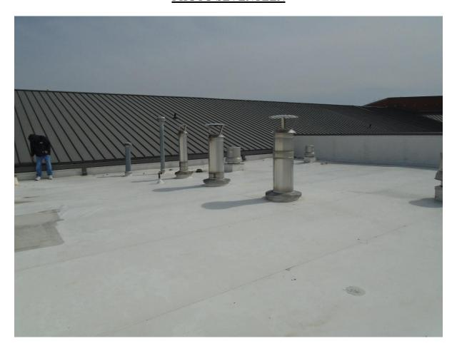
An overview of the Mechanically Attached Thermoplastic Roof **CONDITION:** System on Section C.
