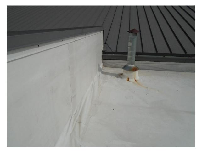
**CONDITION:** The sheet metal cap is rusted at this location.
