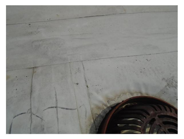
**CONDITION:** The field membrane is cracking at this location.
