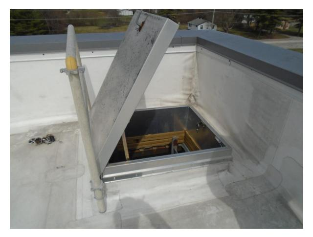
**CONDITION:** Roof traffic around the roof hatch presents a fall hazard. A safety rail system should be installed along this perimeter.
