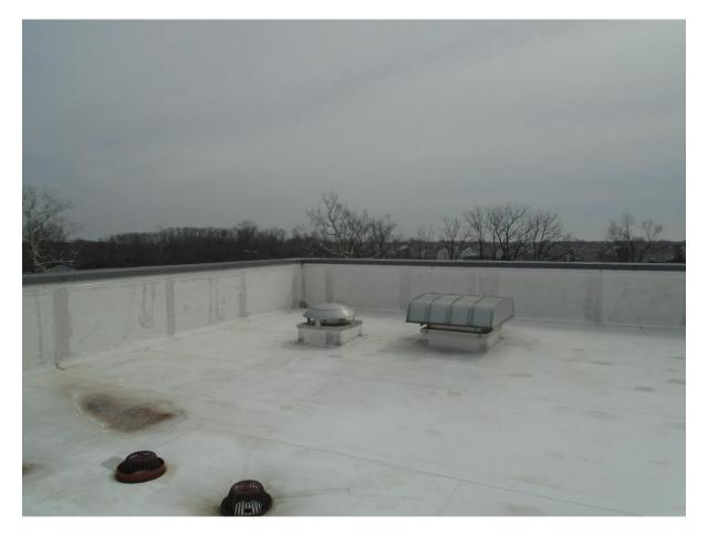
**CONDITION:** A view of wet substrate identified in the Infrared Roof Moisture Survey; no surface anomalies were identified in this area.
