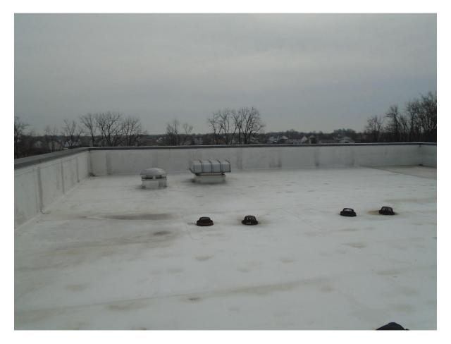
CONDITION: An overview of the Mechanically Attached Thermoplastic Roof System on Section D.
