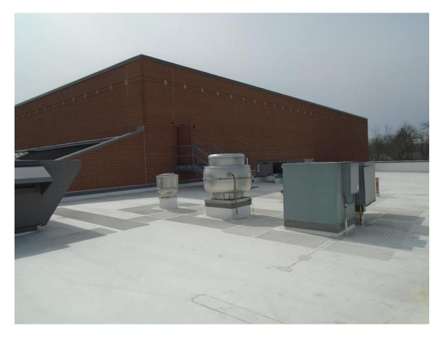
**CONDITION:** An overview of the Mechanically Attached Thermoplastic Roof System on Section B.
