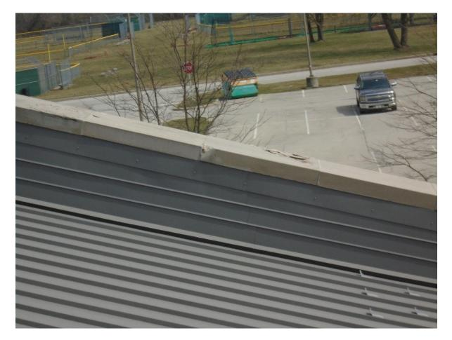
**CONDITION:** The masonry coping stones are deteriorating at this location.
