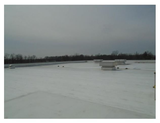
**CONDITION:** An overview of the Mechanically Attached Thermoplastic Roof System on Section A.
