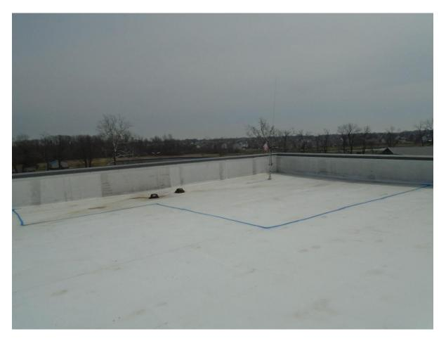
**CONDITION:** A view of wet substrate identified in the Infrared Roof Moisture Survey; several surface anomalies were identified in this area.
